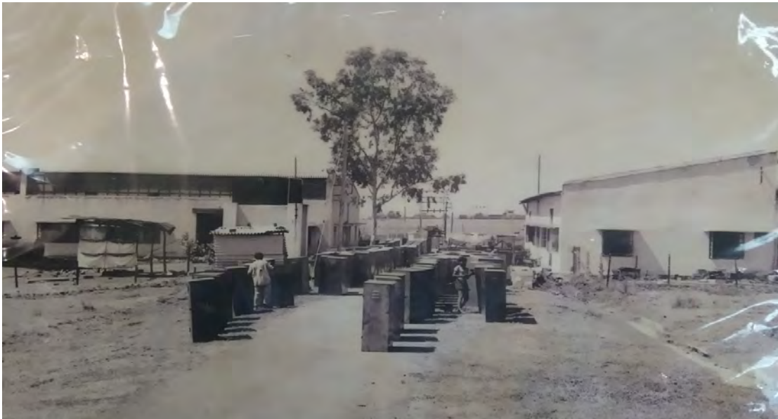
Decades back initial phase of above Manufacturing Facility as setup by Late Shiv Kumar Jhalani (Stock of Distribution Boxes)
